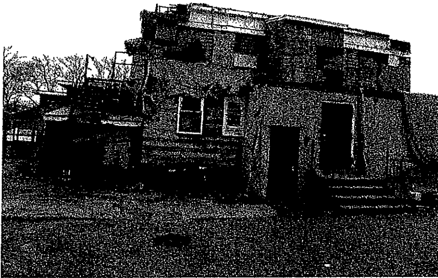
Photograph # 1 – Rear elevation of the subject building
