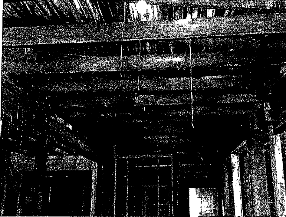
Photograph # 6 – Interior roof framing over the slab on grade section of the building at the front of the building
